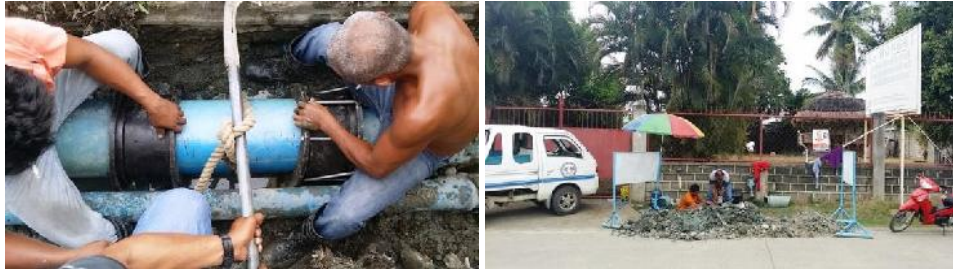
19. Vito 40 HP/460V Pull-out and replacement of 25HP/230V Submersible Pump and Reconfigured the Generator back from 460V to 230V
