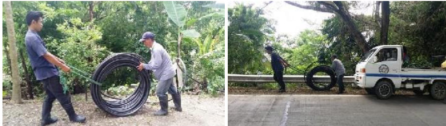
30. Pipe Laying of 2" PE Pipe in Syntech Properties located in Pondol, Balamban, cebu.
