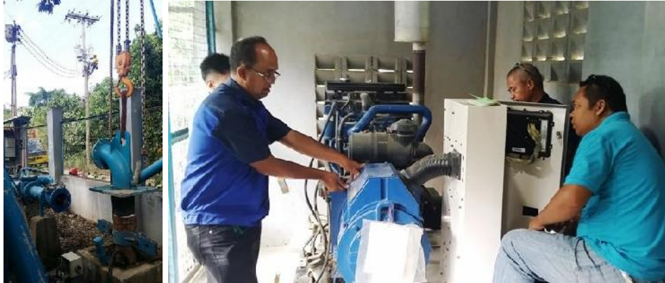
20. Upgrading of Pumphouse in Suron, Hingatmonan Spring.
