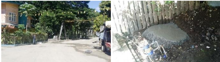
29. Pipe laying of 1200 LM, 1" PE Pipe at Guya, Prenza LGU-funded.
