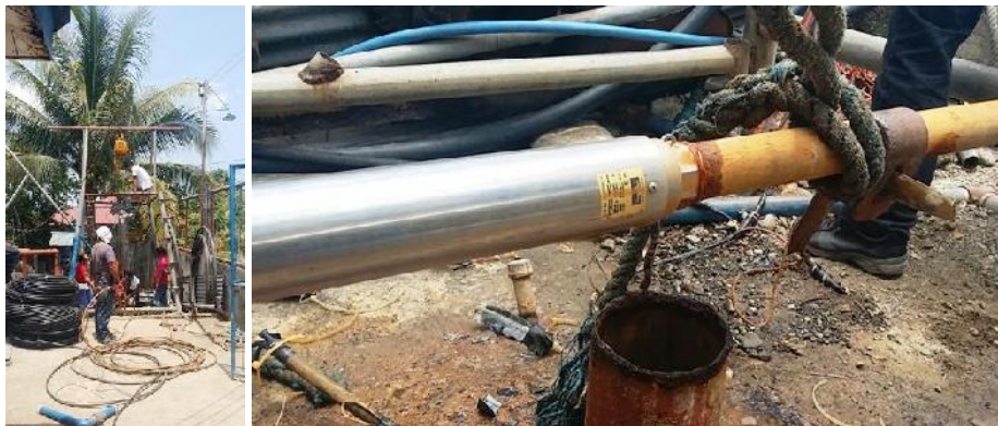
21. Pull-out and Replacement of 7.5 HP, submersible pump in Upper lamak pumping station in Pondol, Balamban, Cebu.
