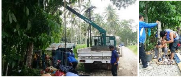
28. Installation of Booster Pump in Pitogo, Hingatmonan, Cebu.
