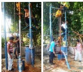
31. Pull-out and Replacement of 7.5 HP, submersible pump in Lower lamak pumping station in Pondol, Balamban, Cebu.
